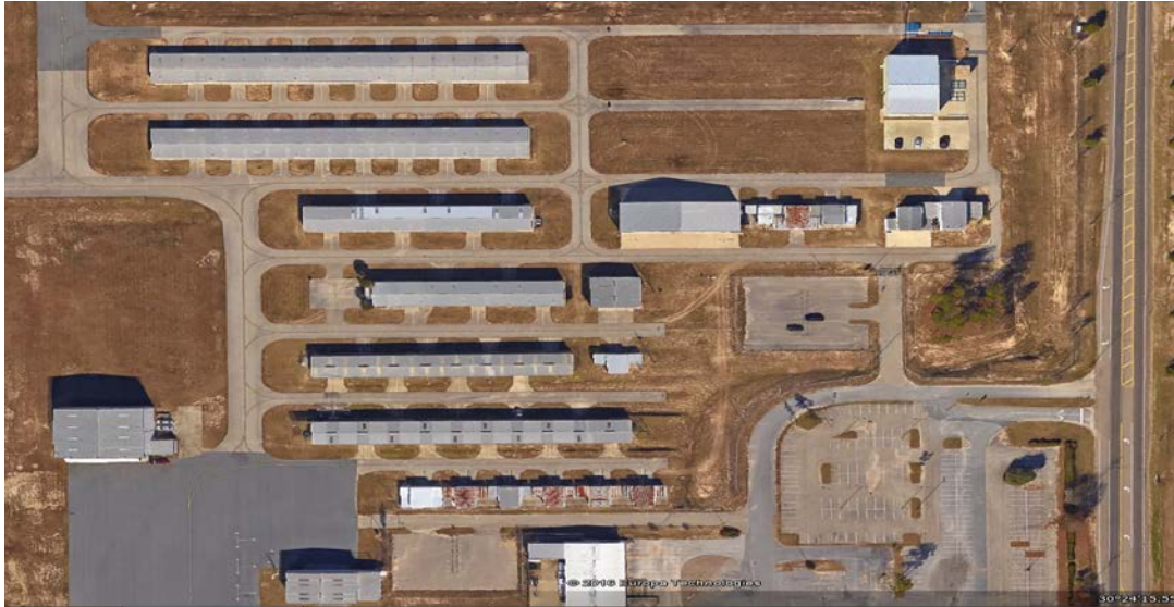
Image 1: Aerial Photo of the Flightline T-Hangar Complex
